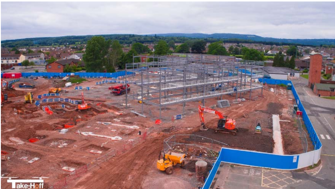
Ariel view – New Caldicot School in construction.
